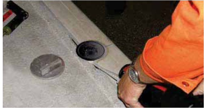
Seal the groove with sealant and adhesives Installation
