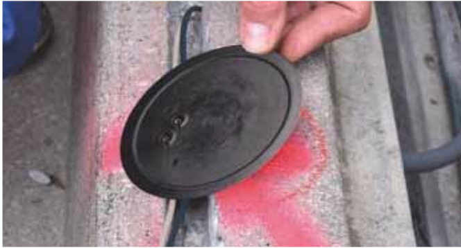
The current collector is installed over the stranded wires
