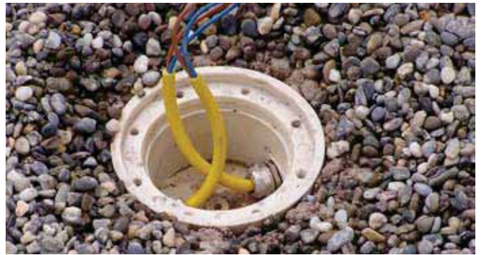
Fill in suitable material around the lower part of the CircLED®
