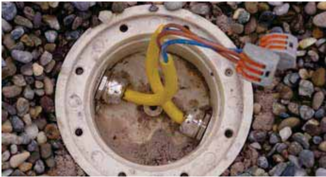
Properly attached connecting clamps
