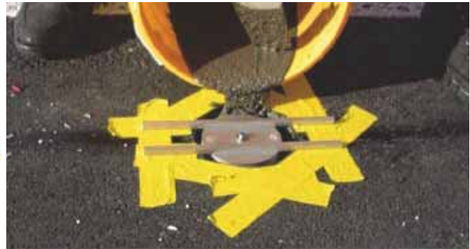
Molding with 2-K mortar
