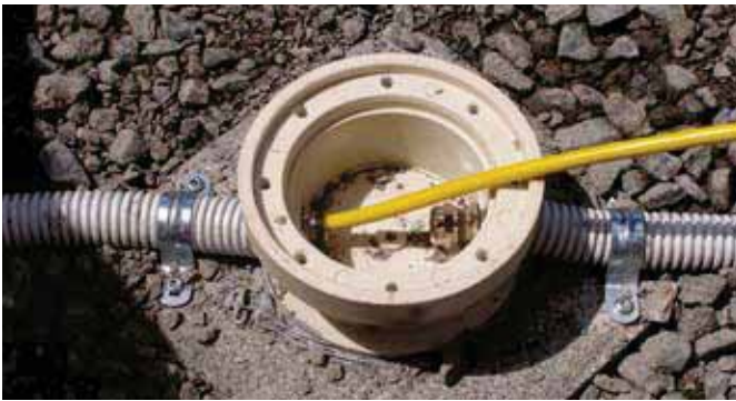
Setting the lower part of the CircLED® in the soil / cable conduit
